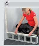
Apply Block Lock glue on a horizontal profile and place it over the first layer of glass blocks.
