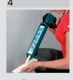
Apply Block Lock glue on a vertical 18 cm profile on both sides
