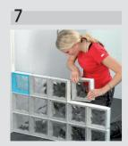
Continue with the next layer. Assemble 5-6 layers and leave them to dry. Continue with assembly after 24 hours.
