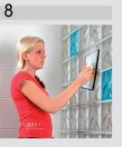
After the wall has dried for approximately another 24 hours, grout the joints with Block Lock glass block grout in any colour of your choice.
